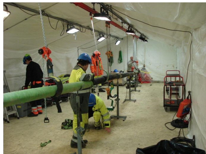
Figure 2 - Repair work on HVDC cable: Moyle Interconnector
